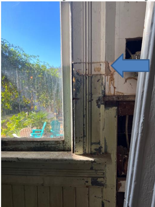
Interior window showing the amount of counter coverage.
