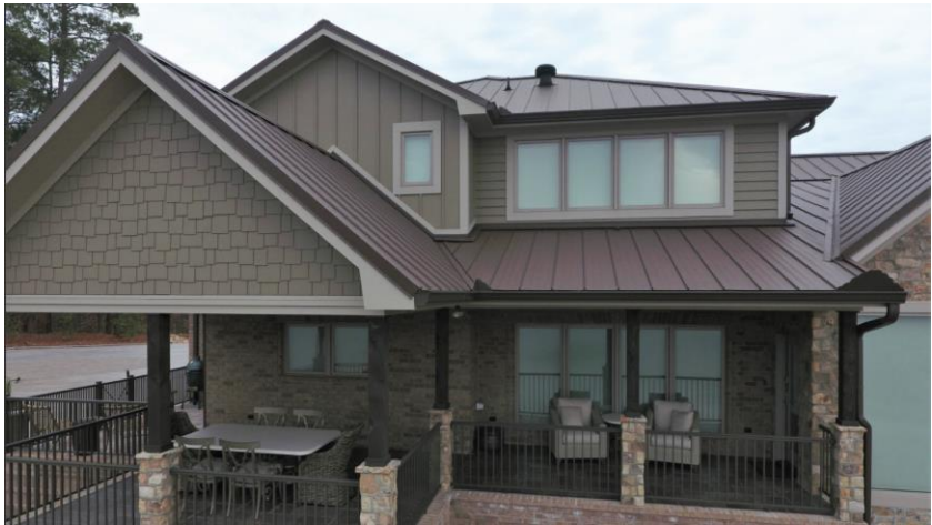
Example: Snap-lock standing seam roof system
