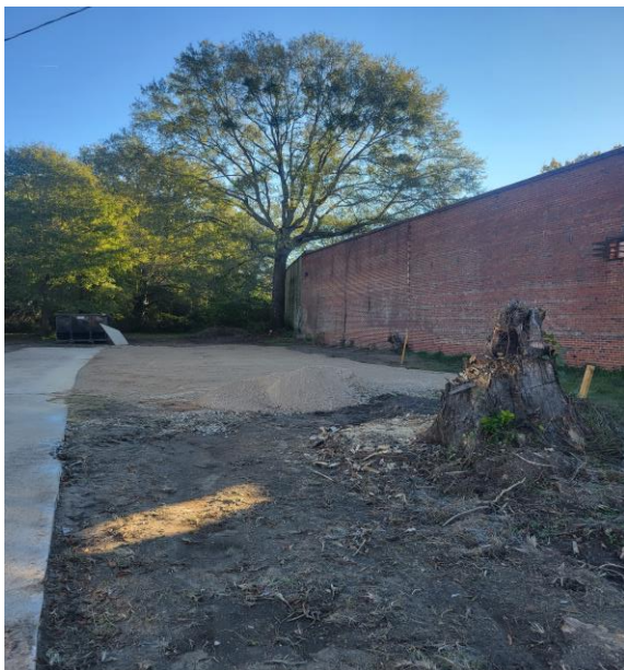
Shed has been demolished and site prepped for parking area.
