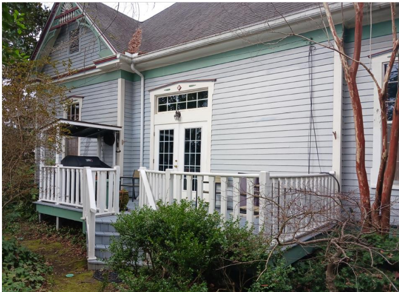
Existing side deck
