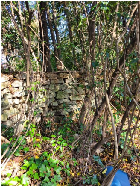
Stone wall at rear
