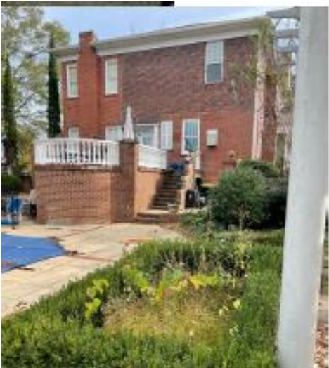
Rear view of house/yard
