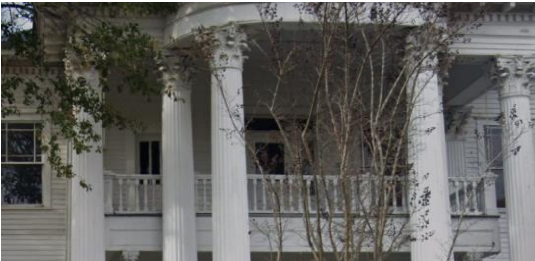
Second floor single door on left to be removed. Interior space to become bathroom. The center single door to be changed to double wood door unit to match front door.
