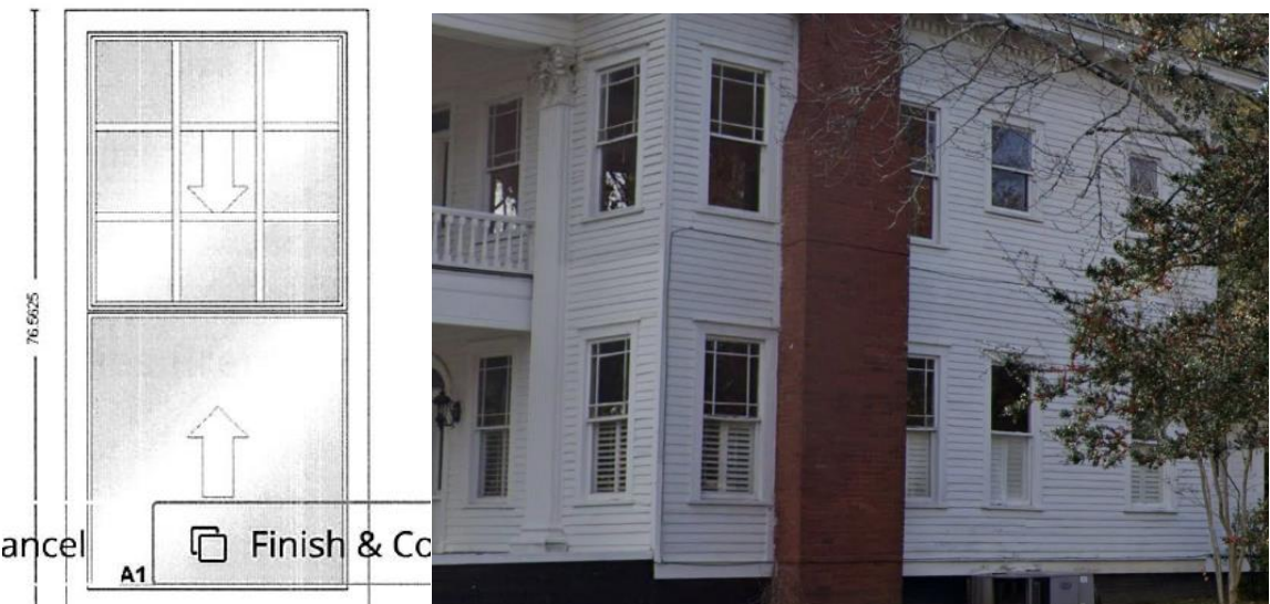
MO 37 13/16" x 76 3/4" AmerCraft Alum/Wood with exterior grids. Photo of Current window patterns.
