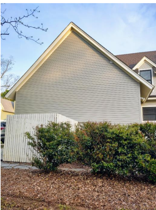
Window location from side yard
