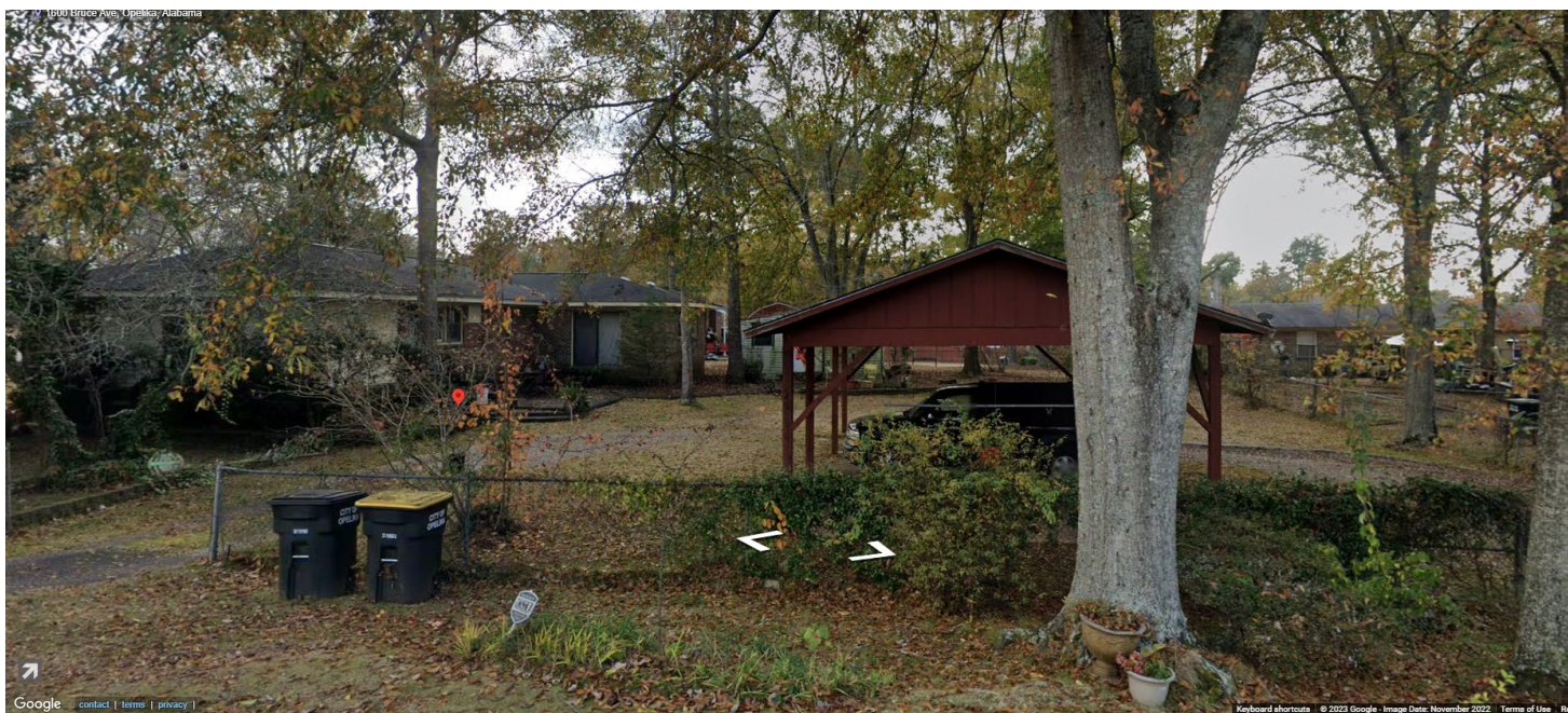
1600 Jollit Avenue - Photo from Bruce Avenue, Rear yard area
