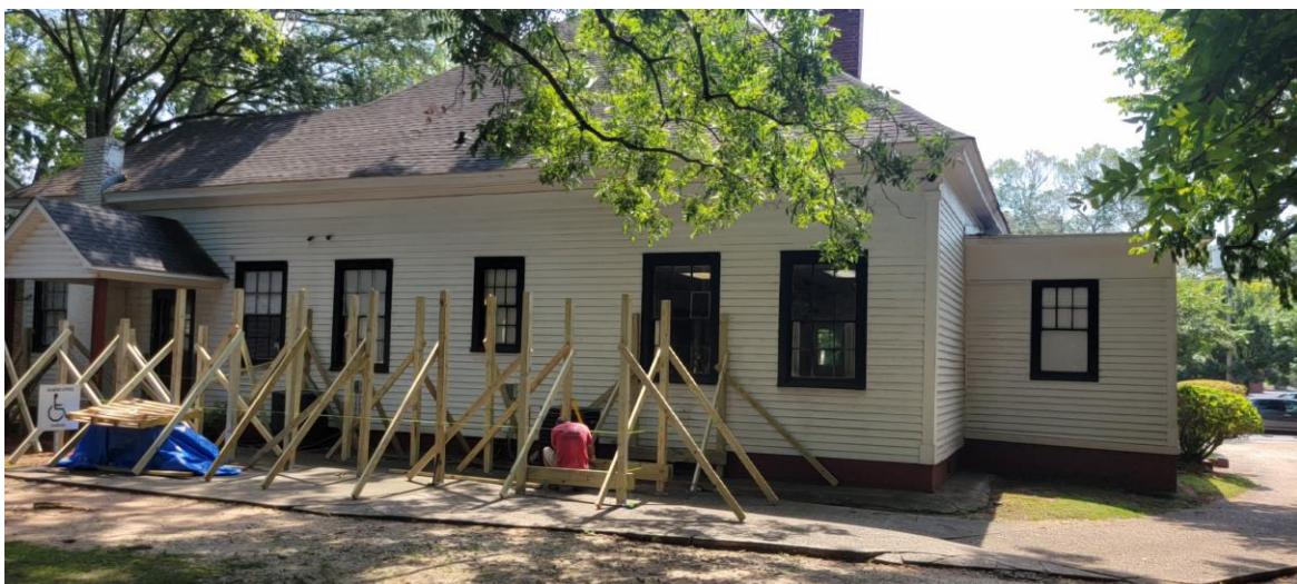
Rear- (5) 6/6; Two windows are being converted to entryways
