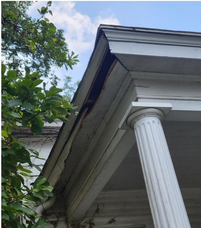
Additional damage by fallen tree to be repaired (with internal gutter system)
