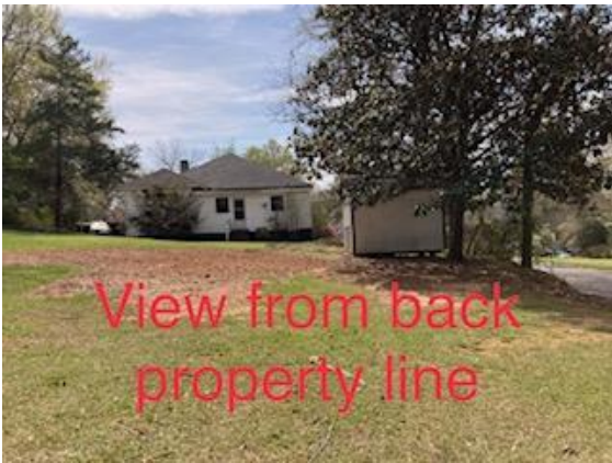
View from back property line
