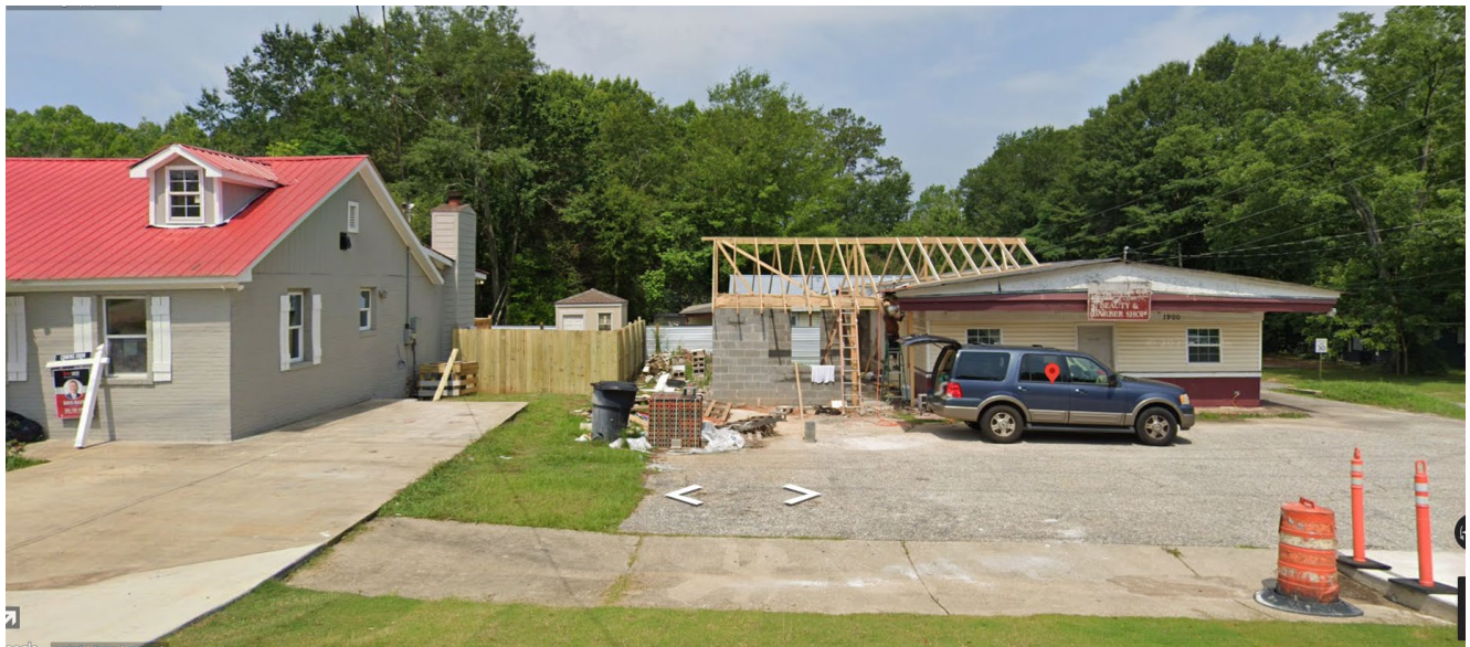
8x10 addition under construction. Photo taken from South Long Street
