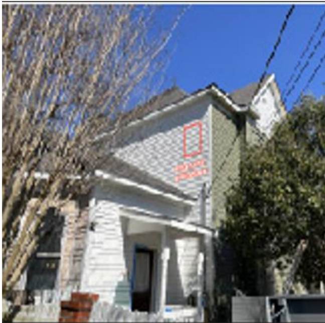
Location of window on 2 nd floor; rear of home
