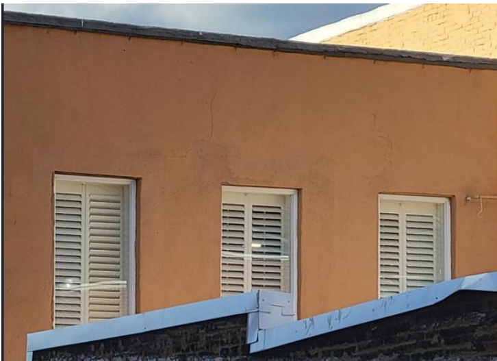
Rear windows- exterior view
