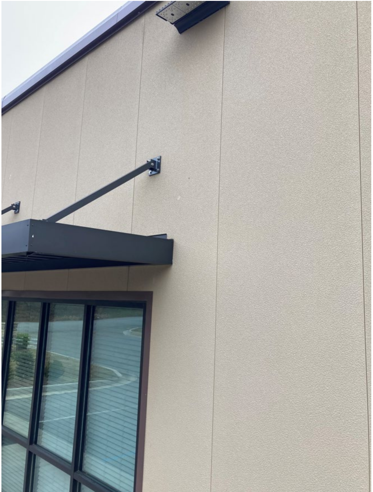
Example of similar metal architectural panel with a stucco like finish provided by the applicant.
