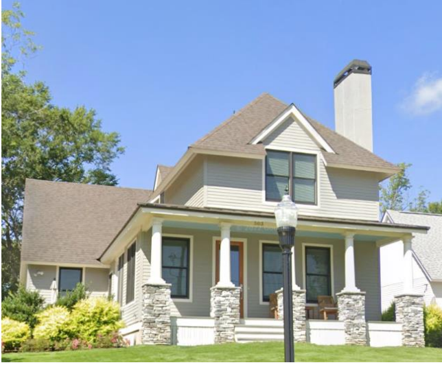
New construction w/rock column foundation
