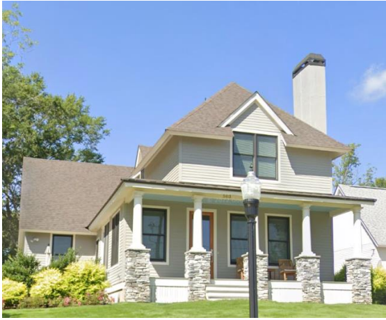
S. 8 th St-New Construction
