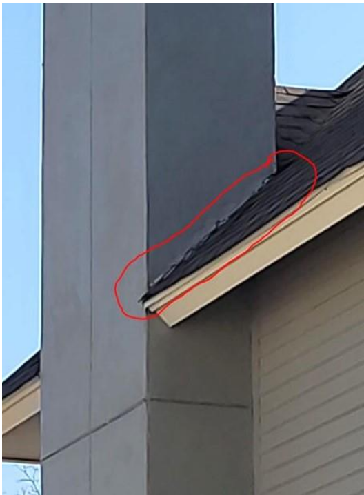
West side flashing
