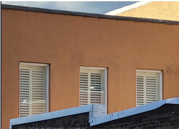
Rear windows- exterior view
