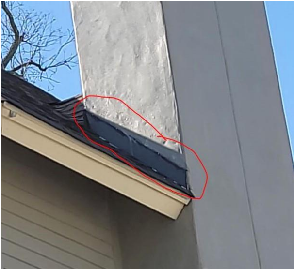
East side flashing with extra patch
