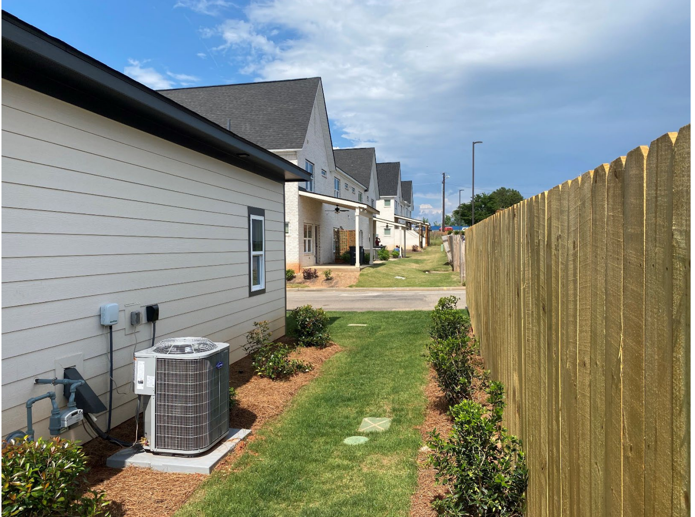
Portion of Rear wall of one-story units 1 to 4 setback 10 feet. In background is taller 2-story units that are setback 20 feet.
