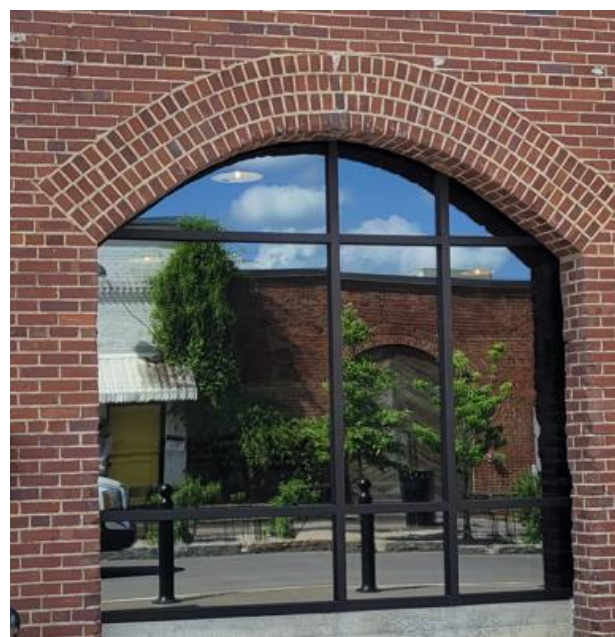
Metal framed windows
