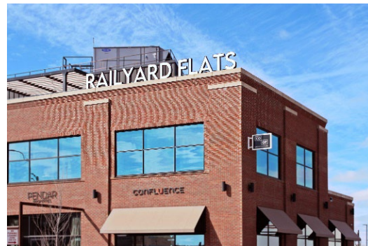
Sign on flat roof.
