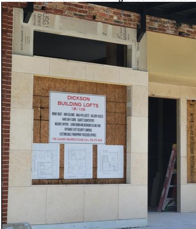
Jerusalem stone tile installed
