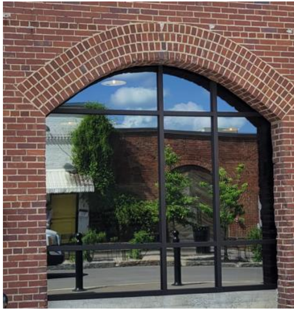
Example of metal framed windows-Resting Pulse
