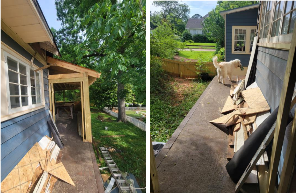
Side porch-new handrails to be installed
