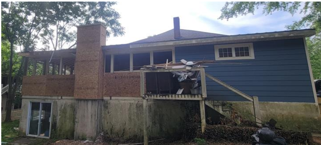
Rear view of extended/enclosed porch
