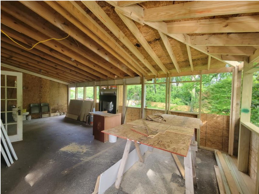
Interior view showing enclosure and new fireplace
