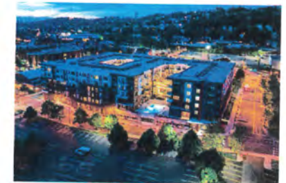
Connection At Southside Pittsburgh, PA
