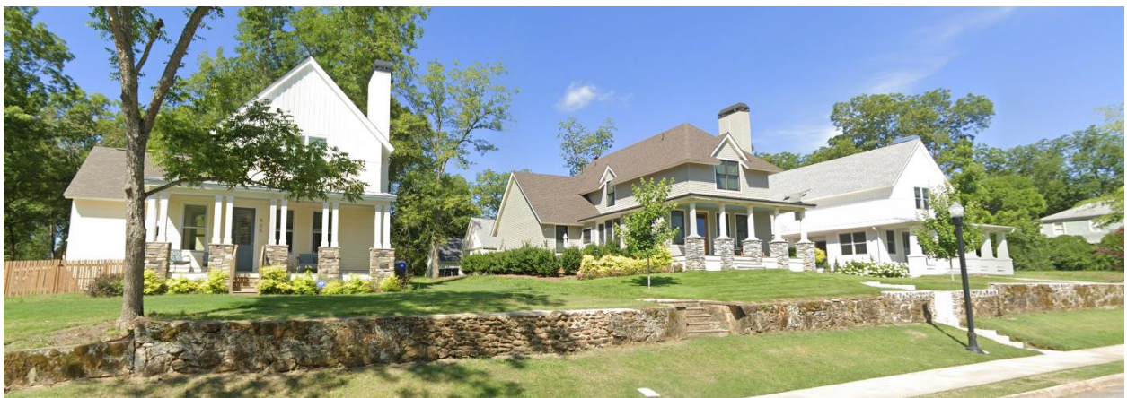
Existing rock and concrete wall with stairs
