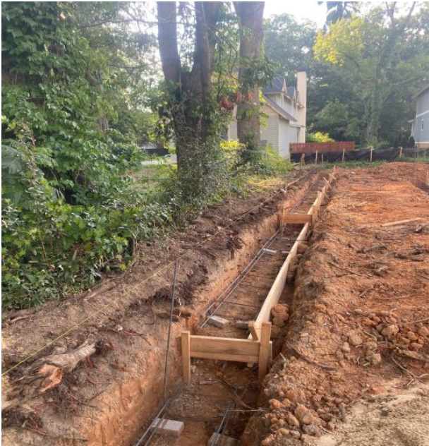
Footing and tree location
