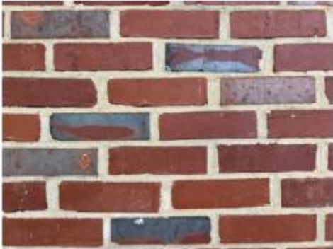
Existing brick on house
