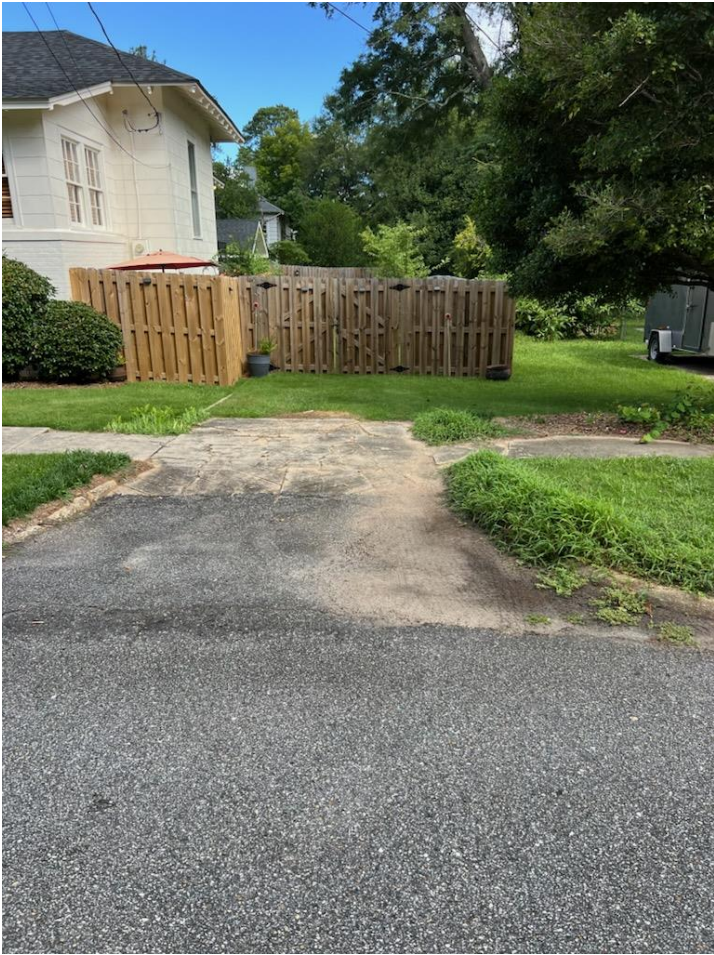
Existing side drive
