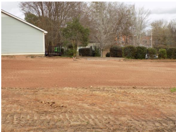
Parking area has been graded and trees Removed as previously approved
