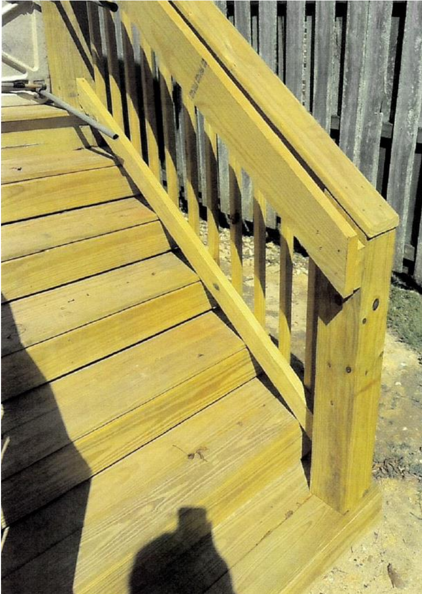
Decking and rail for handicap ramp
