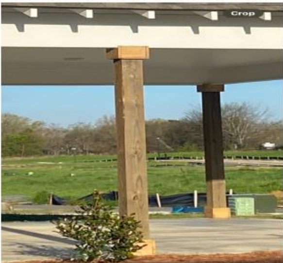
PORCH COLUMNS: treated 6x6 pine columns to be stained or painted to match house
