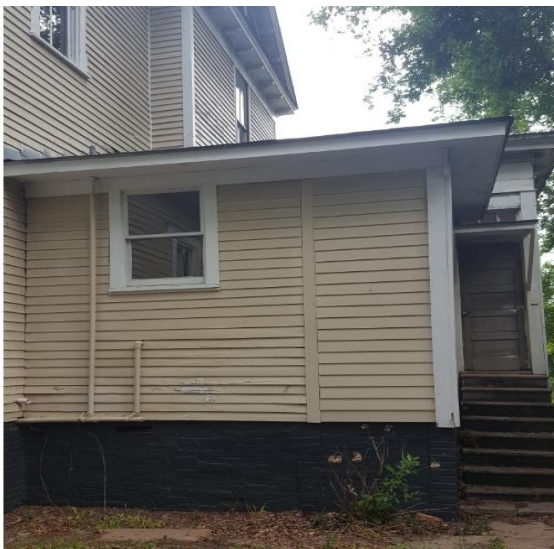
Rear addition to be removed
