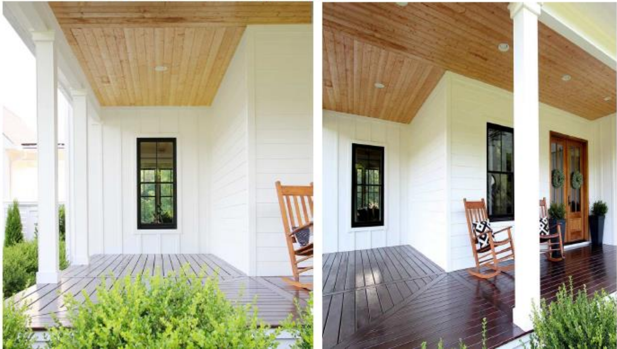
PORCH CEILING: v-groove pine tongue and groove
