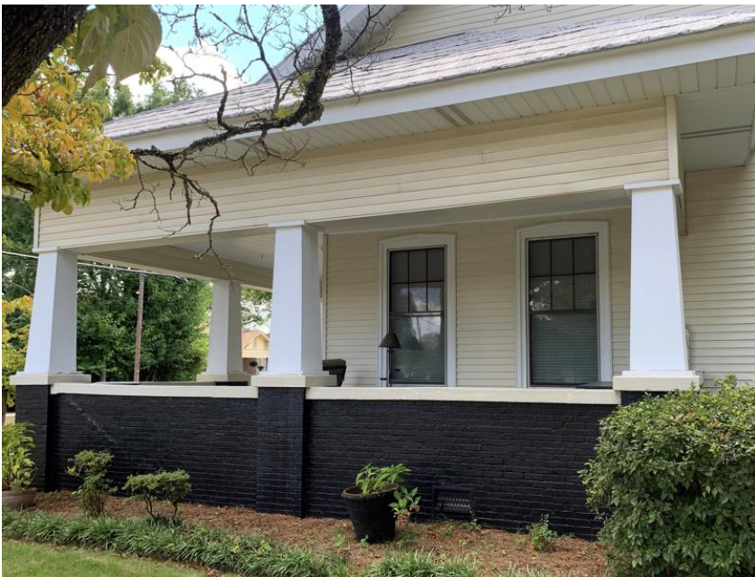
Side of front porch-2 nd window to be removed and door installed
