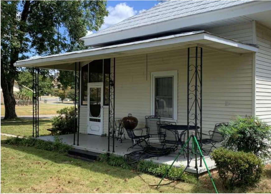
Rear covered porch
