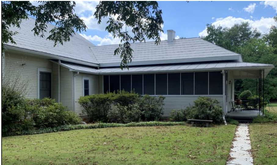
Rear screened and covered porches/walkway from city sidewalk
