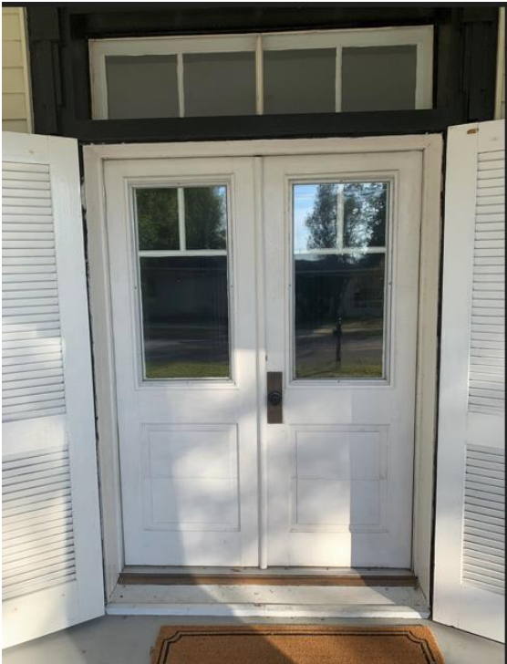
Existing front doors
