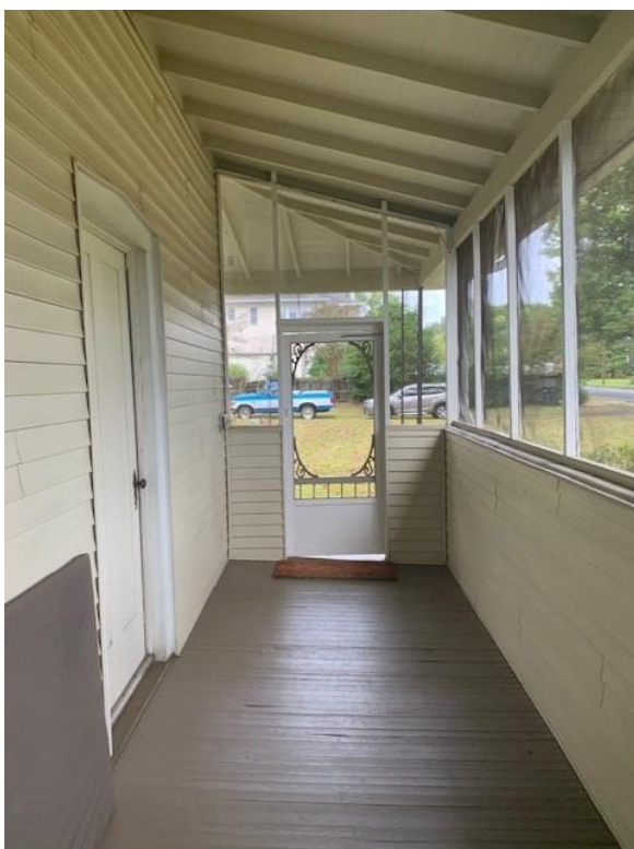
Interior view of rear screened porch with wood floor
