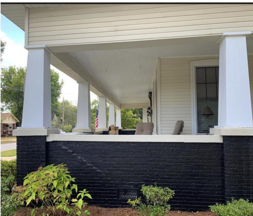
Another view of front porch from side
