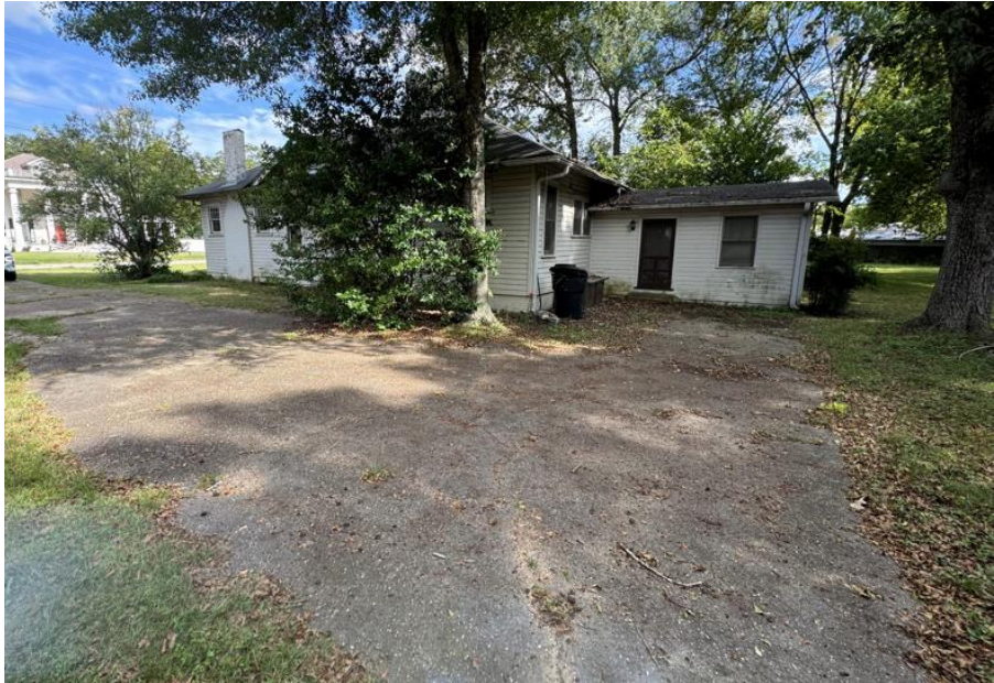
Rear location site for concrete handicap parking pad
