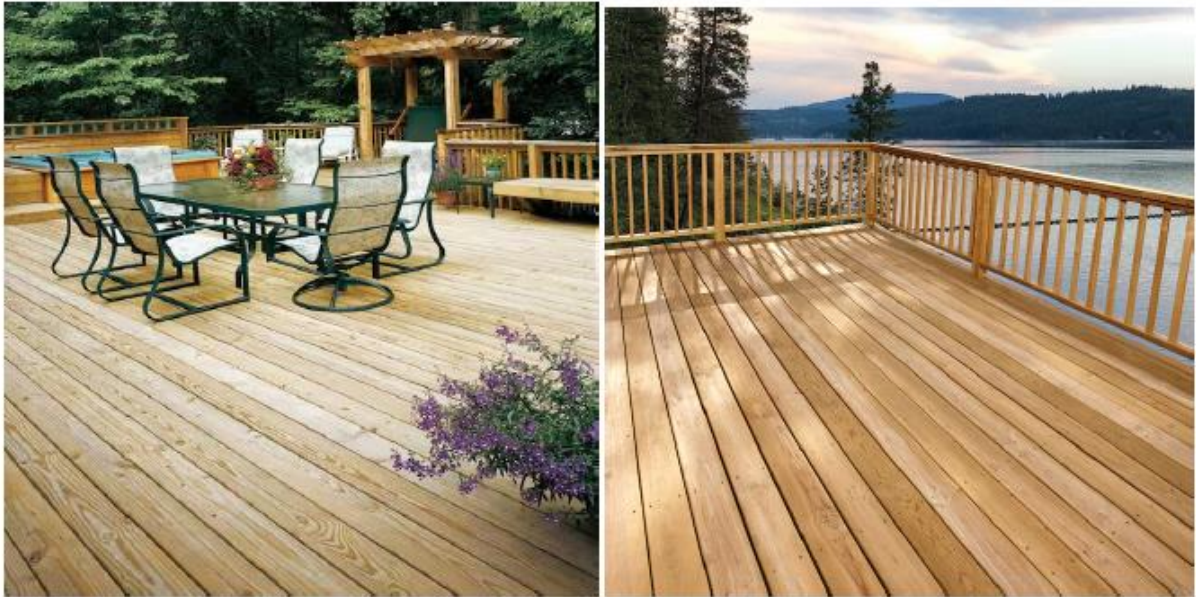
PORCH / PORCH STEPS: 5/4 treated pine deck porch
