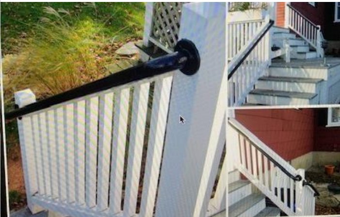
Ex: Wood and Iron handrail
