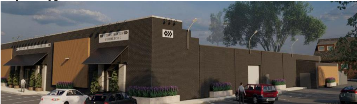
Corner view showing additional gooseneck lights, logo, security lights
