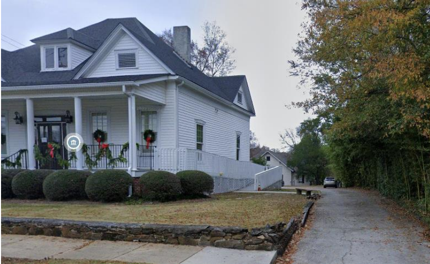
View of ramp from street/sidewalks
