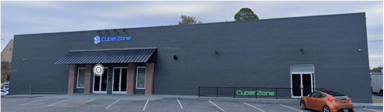
Current front facade
