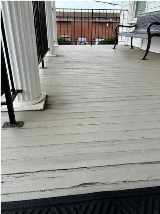
Damaged decking on front porch
