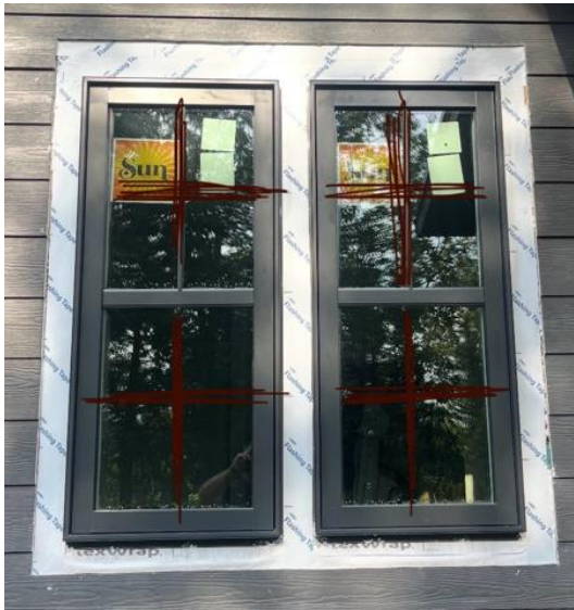
Sun Patriot Series Casement, Fixed Lite out-swinging windows with aluminum exterior and exterior grids as diagramed above which has the appearance of a double hung window. If not allowed, Windor or Pella double hung alum clad windows with 4/4 grids will be installed.
