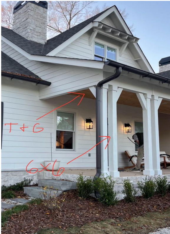
Ex: Porch columns and tongue & groove ceiling
