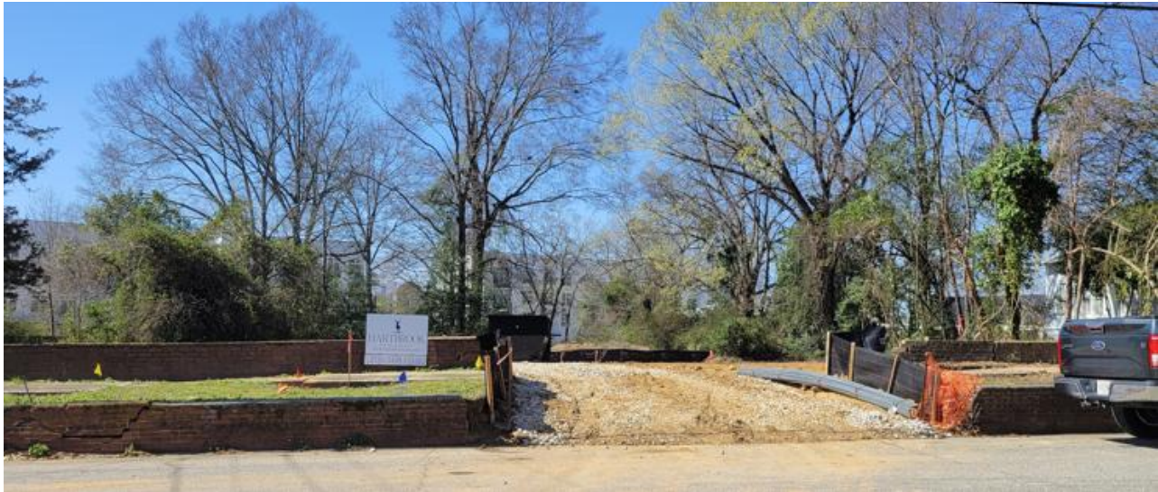
New drive installed for access to twin homes and future development (steps removed)
