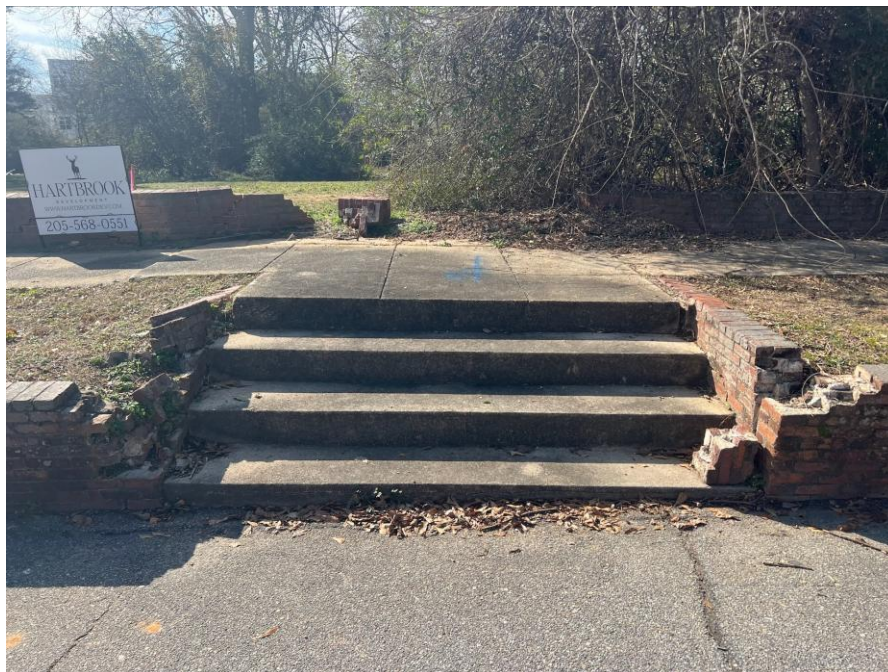
Old concrete stairs
