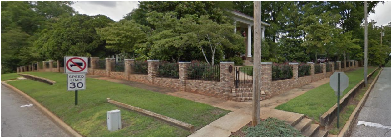
Concrete wall at 4 th Ave/6 th Street
