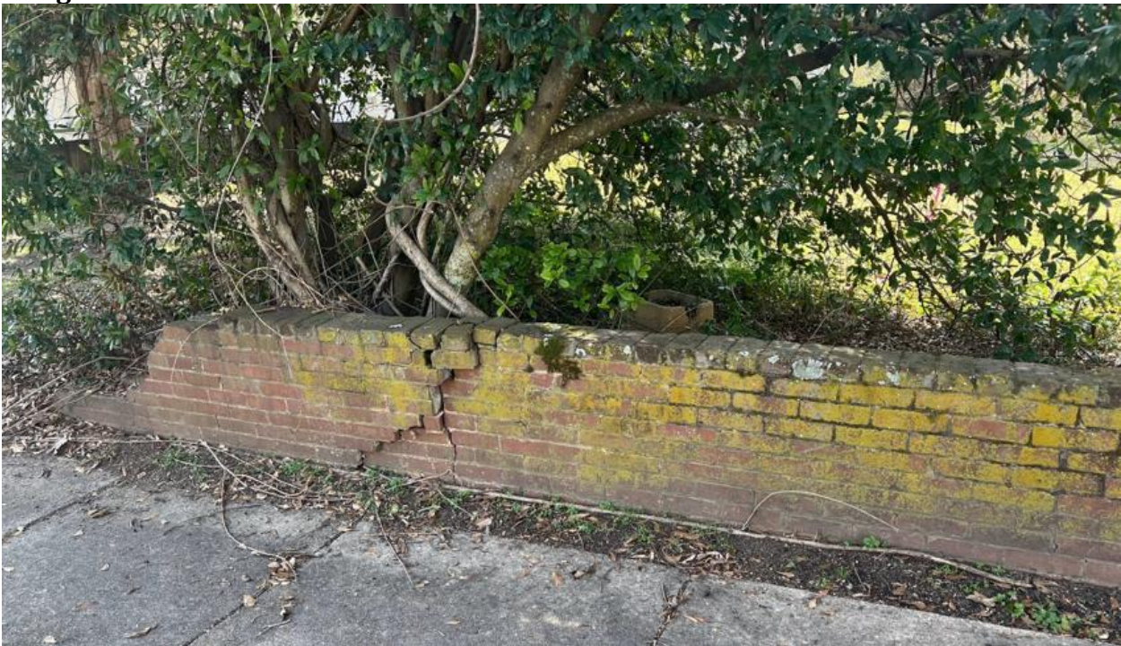
Damaged/failing wall
