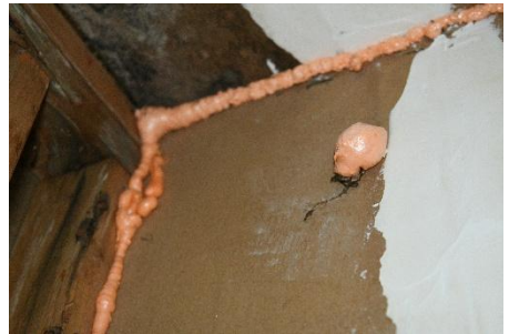
Caulking -Hotel Chase
