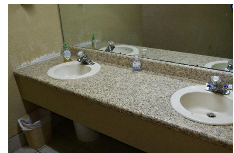
Public Bathroom – Office/Reception
