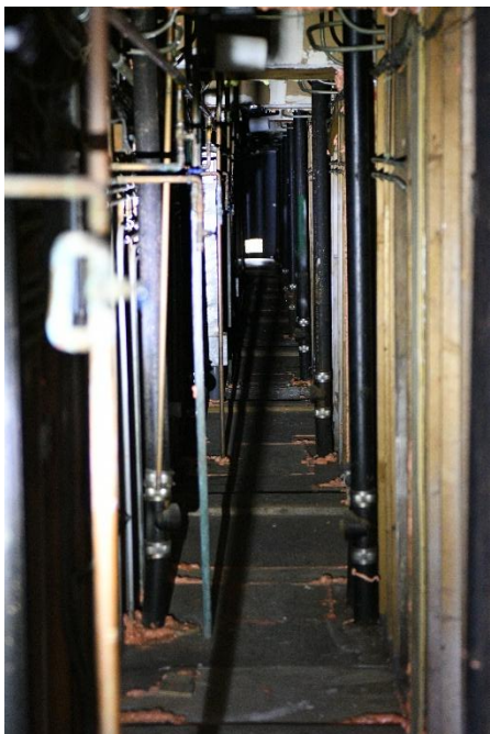
Caulking – Hotel Chase
