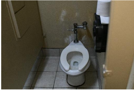
Public Bathroom – Office/Reception
