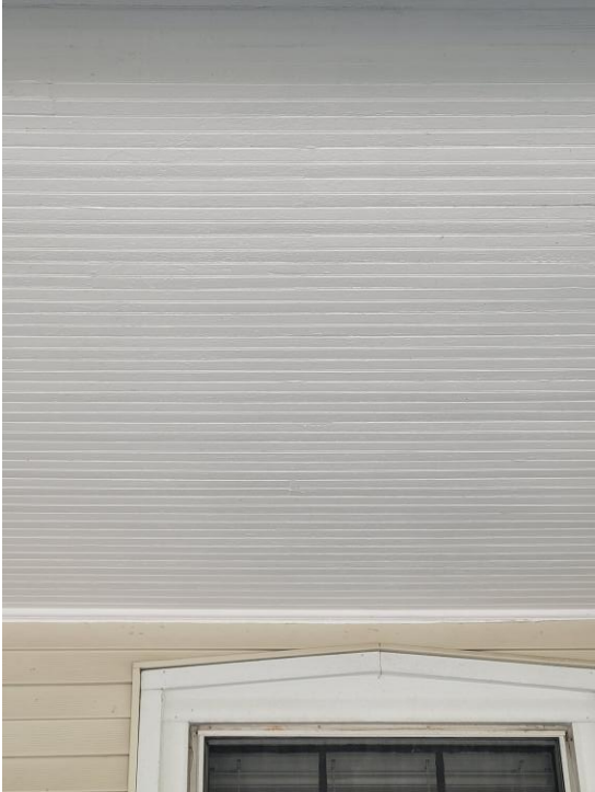
Beadboard ceiling on porch
