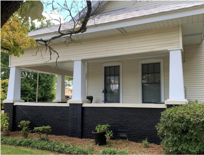
Columns on existing porch
