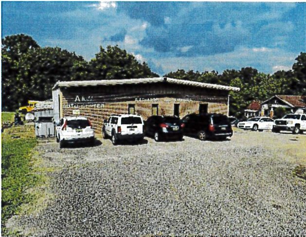
Frontage along S 6 th Street
