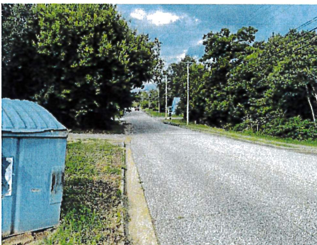
View northeast on Avenue C
