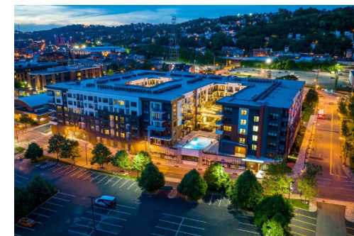
Connection At Southside Pittsburgh, PA
