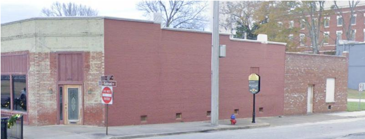
Side view with rear addition
