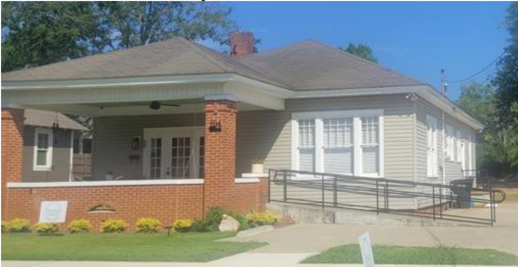
New concrete ramp and parking pad on front of structure
