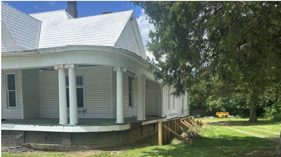
Site of proposed ramp on right side of house
