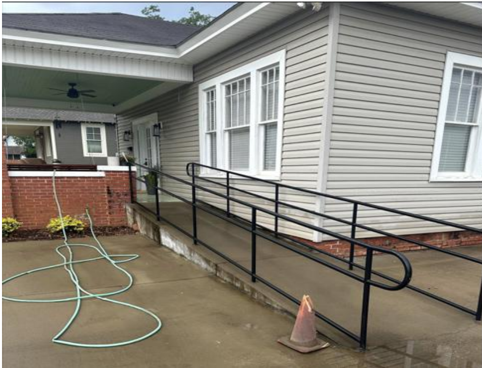
Proposed block and concrete ramp with metal railing
