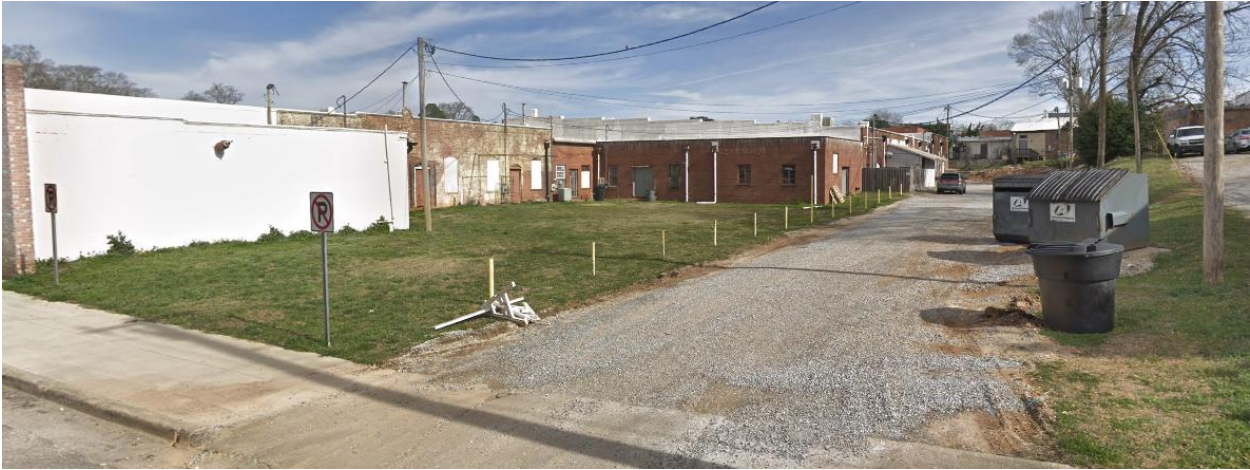
Rear view for courtyard and parking
