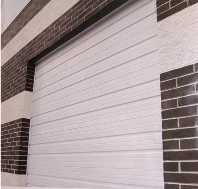
Rear Garage Door
