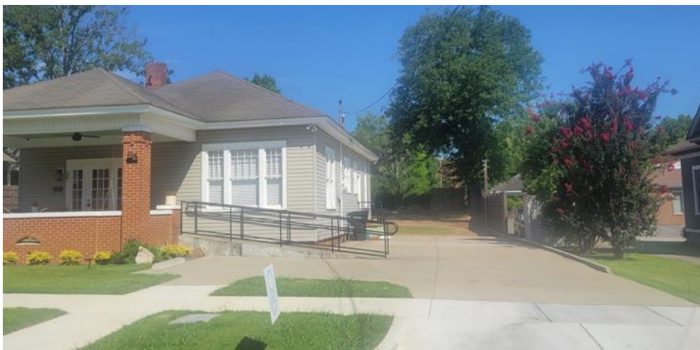
Newly poured concrete driveway without ribbon driveway
