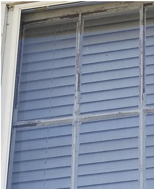
Damaged window/grids
