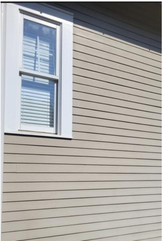
Hardie siding on rear addition
