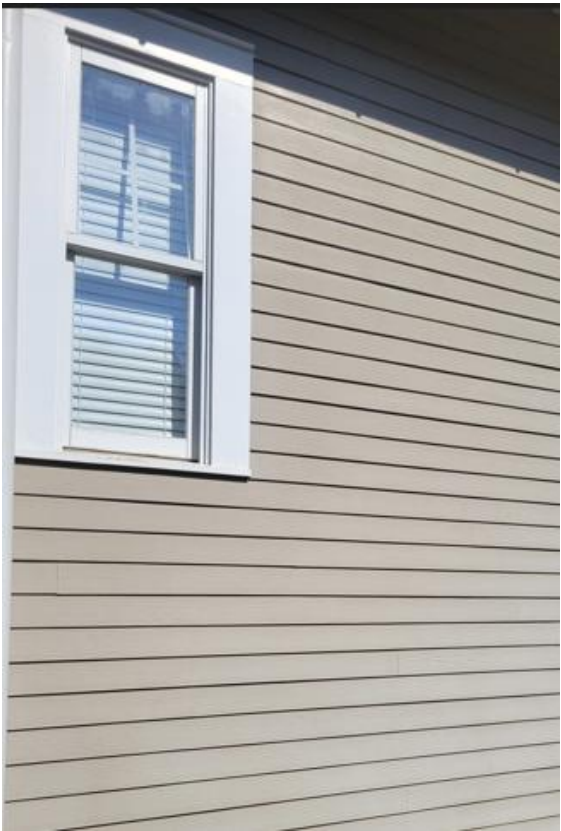
Hardie siding on rear addition
