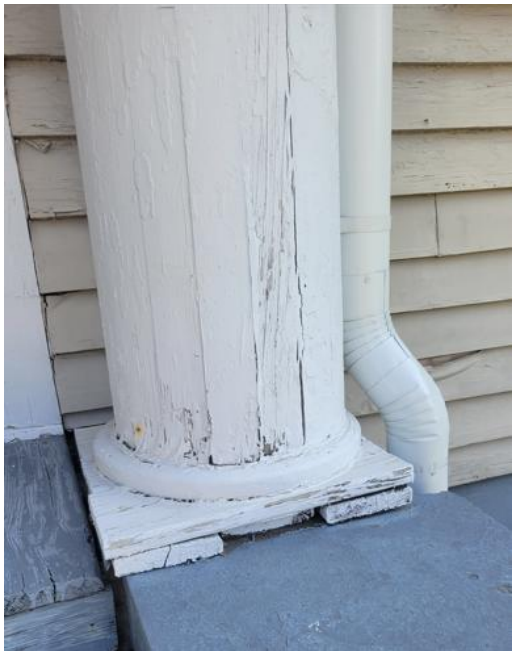
Damaged wood columns
