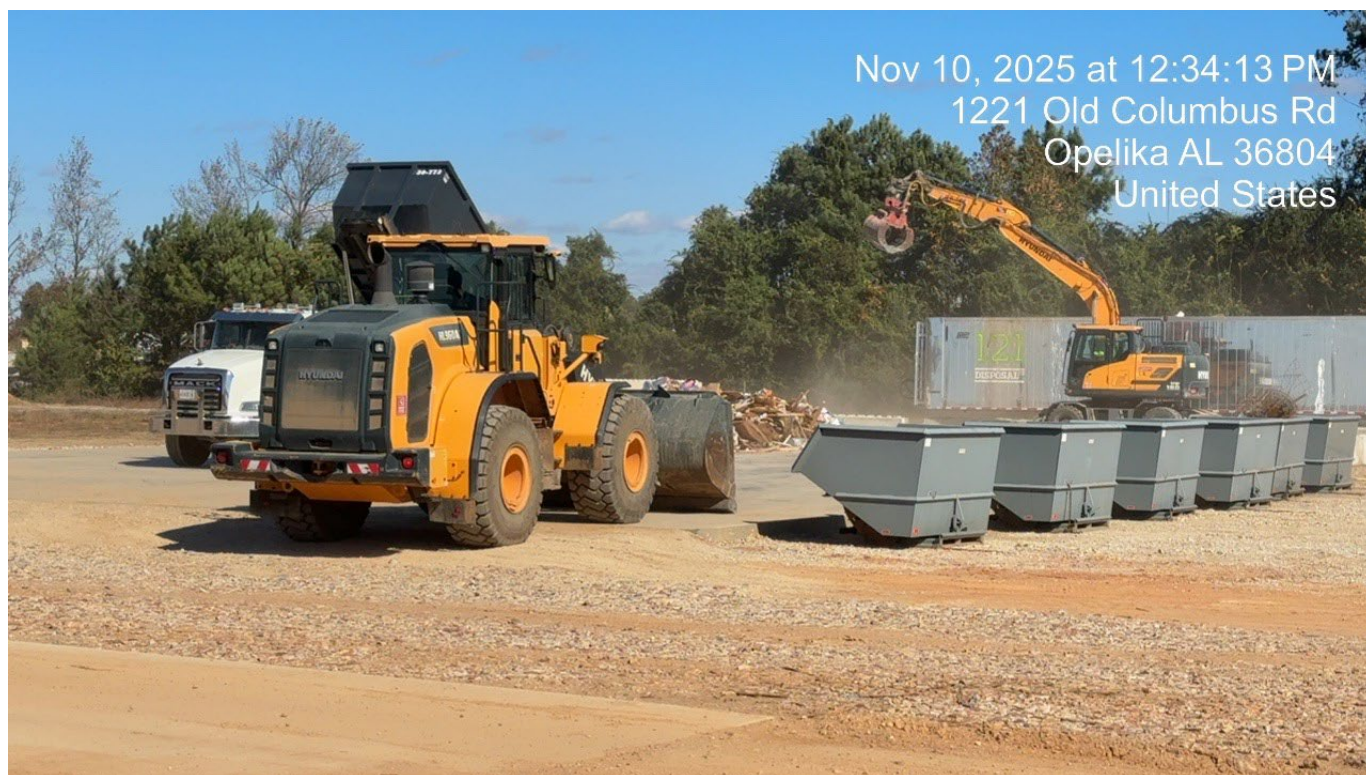
Truck dropping materials and sorting
