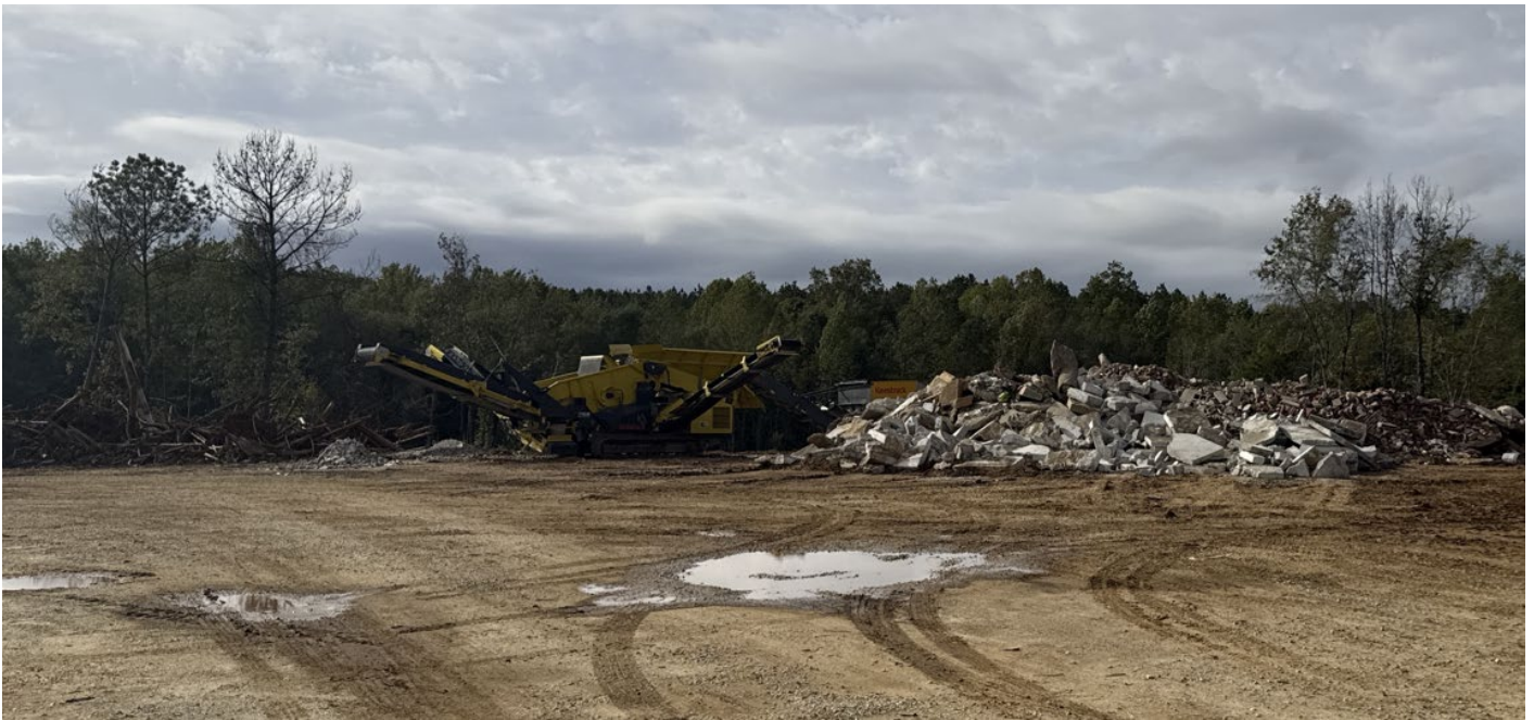
Breaking up concrete
