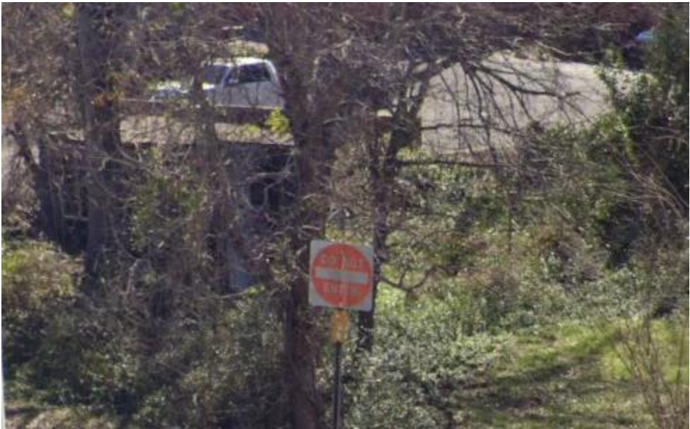
Dilapidated shed in rear of property-remove and clean area
