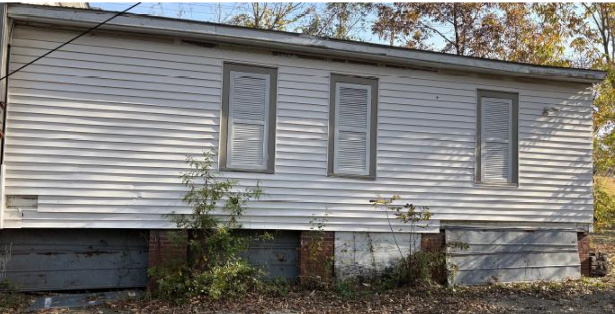
Tin and Wood barricades at crawl space and enclosed with brick
