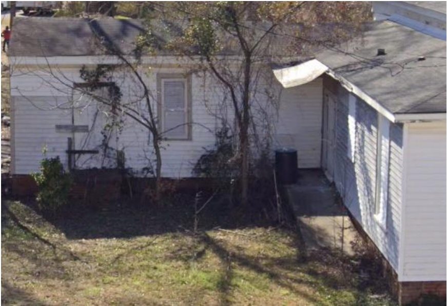
Current concrete ramp on rear
