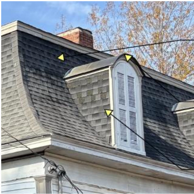
Replace asphalt shingles. Install Hardi on dormers And metal drum caps with standing seam
