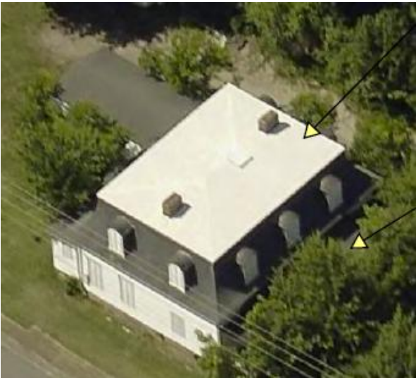
Install new TPO roof on top
