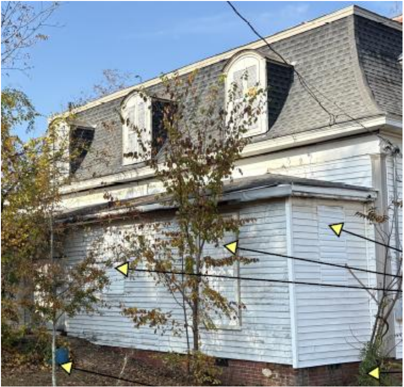
Enclose rear windows to allow for restrooms
