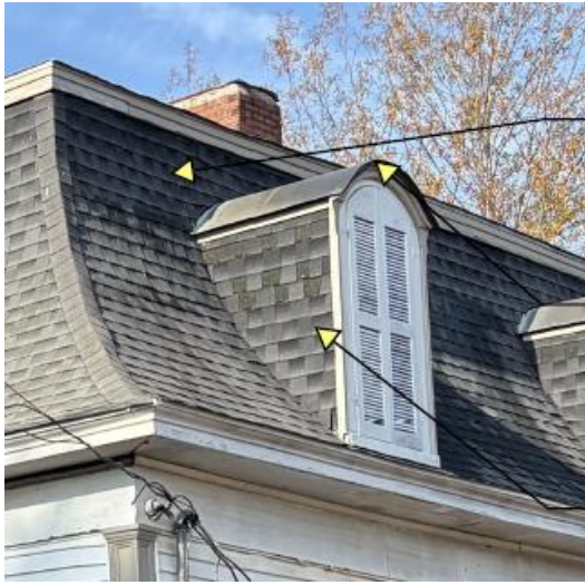
Current asphalt shingle
