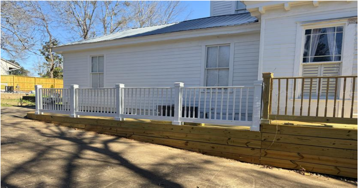
New 10' x 60' deck with ADA ramp
