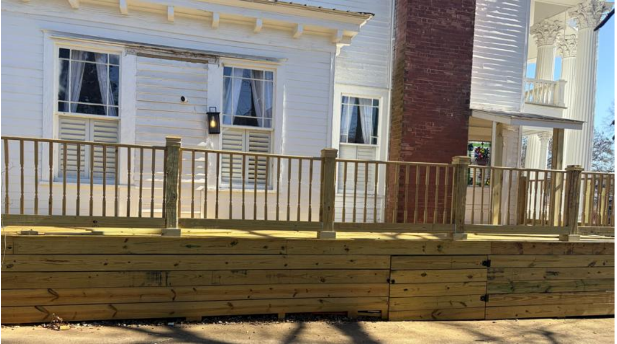
Close view of deck and railing system
