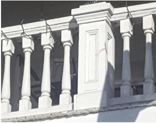
Existing Victorian railing
