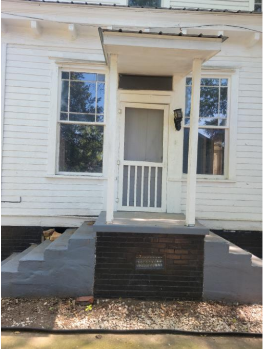
Previous side exit doors and concrete steps
