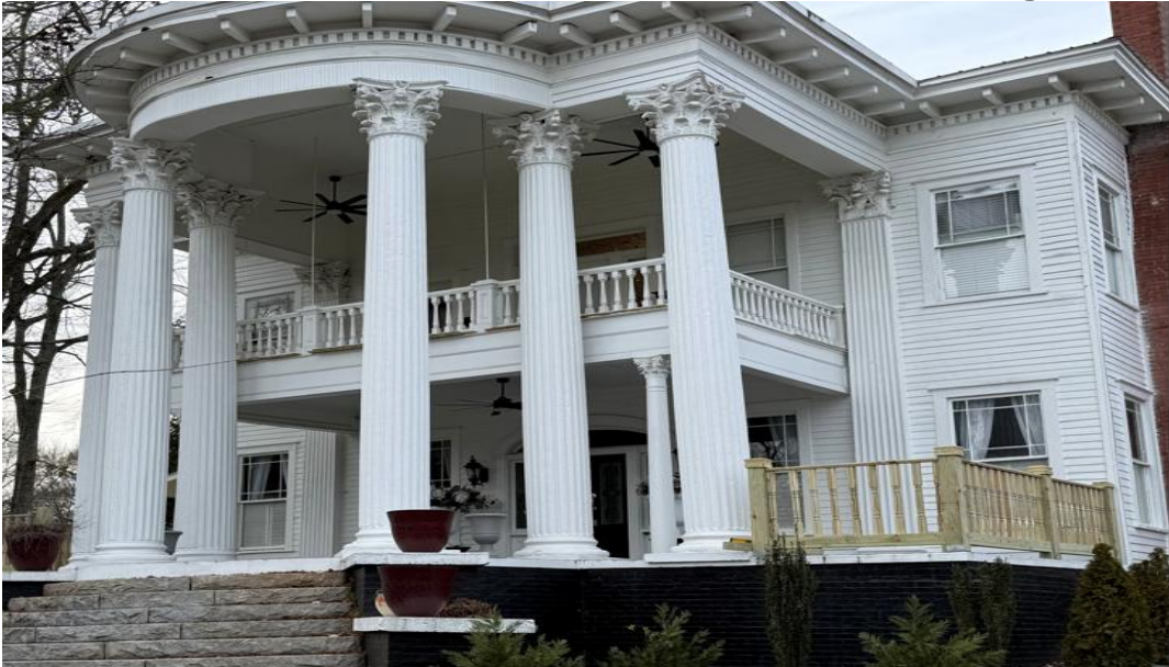
New railing on the right side
