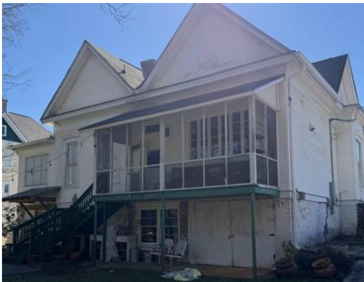
Existing screen porch angled view
