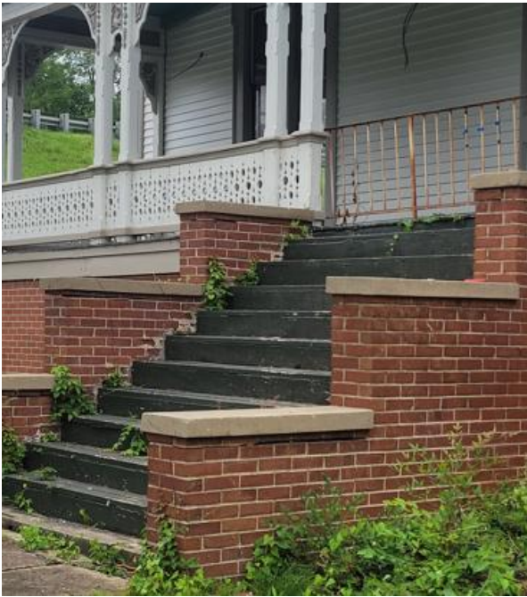
Front brick w/concrete caps
