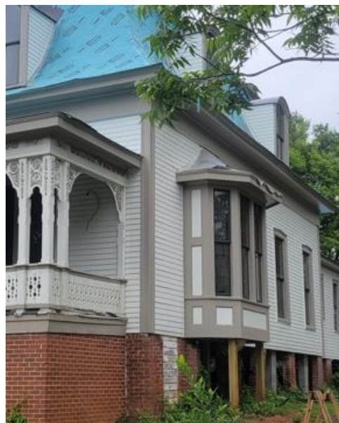
Bay window installed
