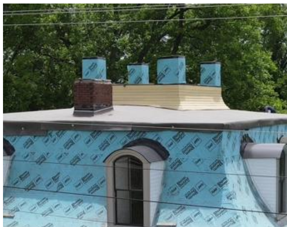
Columns framed and siding base
