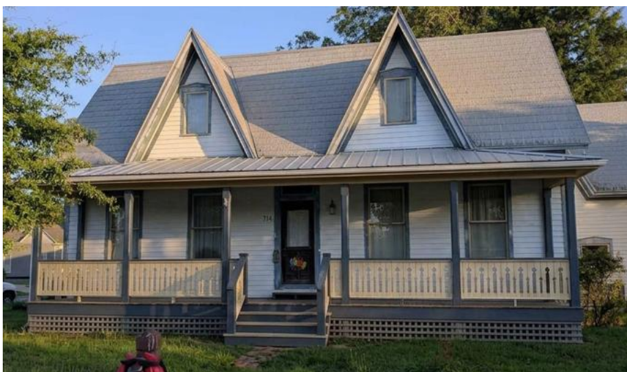
Rendering of porch for front (facing Ave D) to match side porch
