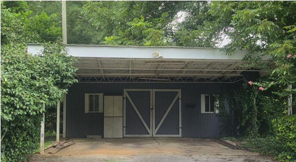
Carport/shed in rear yard- to be demolished to allow addition and parking
