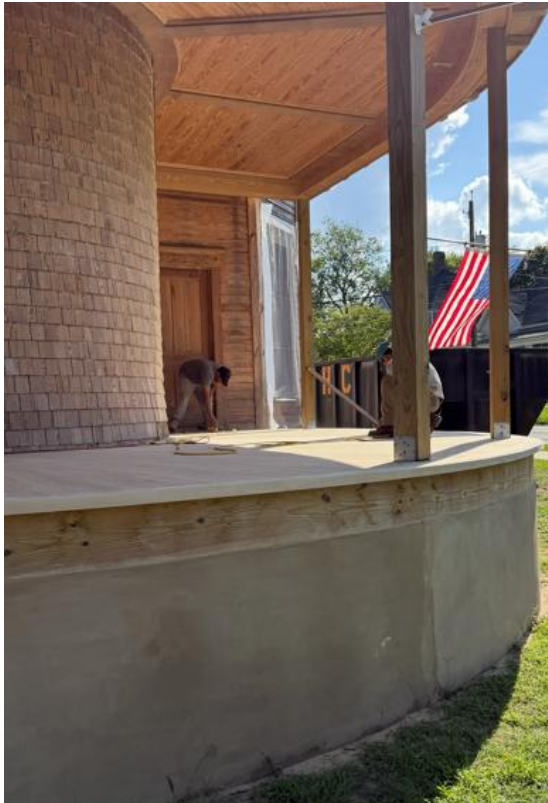
Current house foundation
