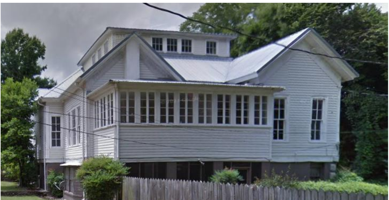
Before rear view
