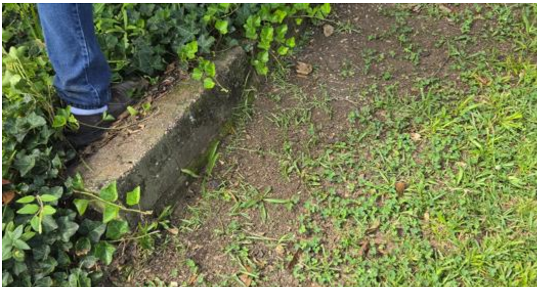
Curb wall will tie into wall on left side along property line
