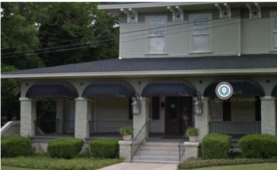
114 N. 11 th St – stone covered with stucco and painted
