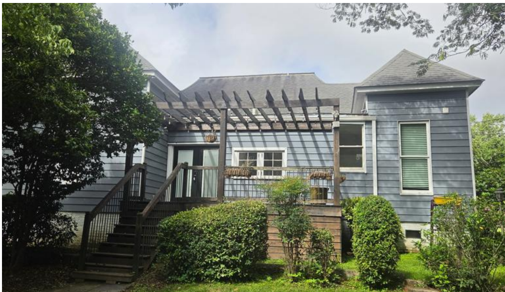
Rear view-deck to be removed and commercial kitchen addition added
