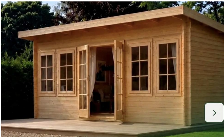
Shed front view with wood lap siding
