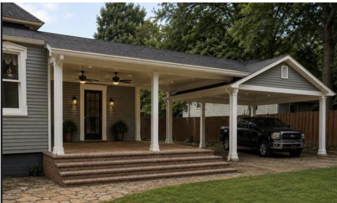
Picture for covered patio and carport
