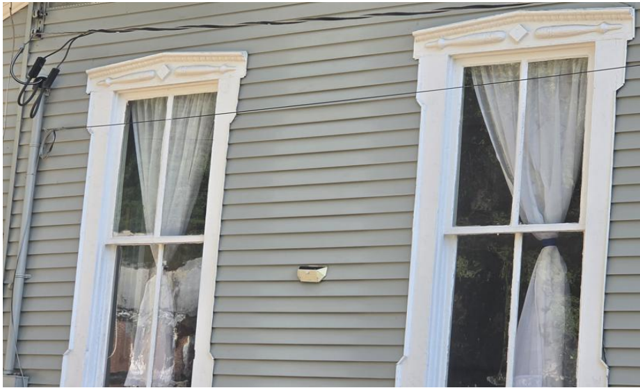
Architectural features on side windows
