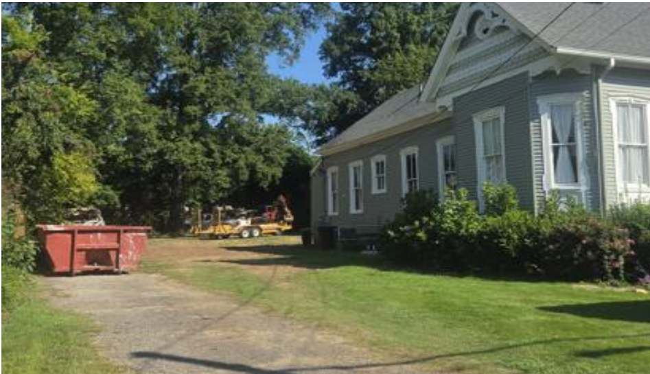
Side yard view for double carport
