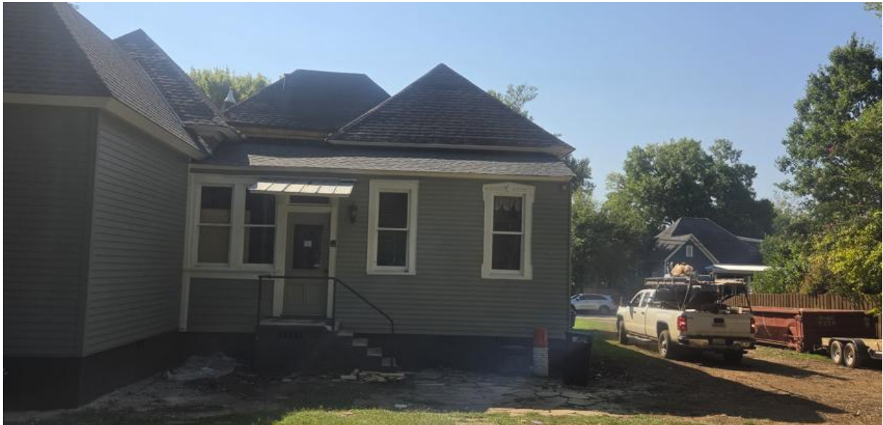
Rear view-current roof line is above windows
