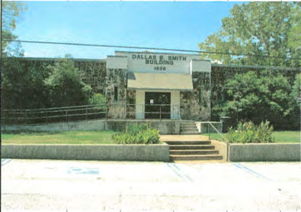
DALLAS B. SMITH BUILDING
