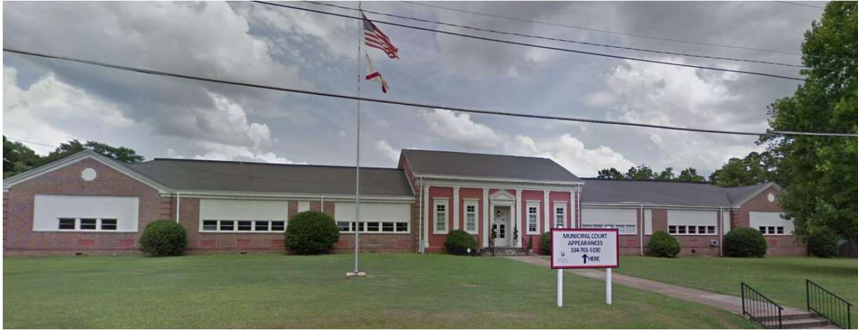
Front of building
