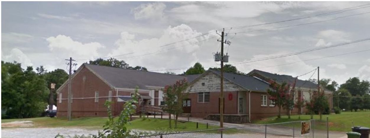
Rear View-retaining wall and circular drive will be installed for drop off at rear entrance.
