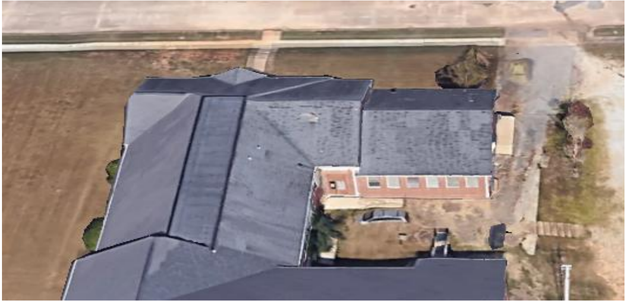
Aerial view of Senior Center Wing
