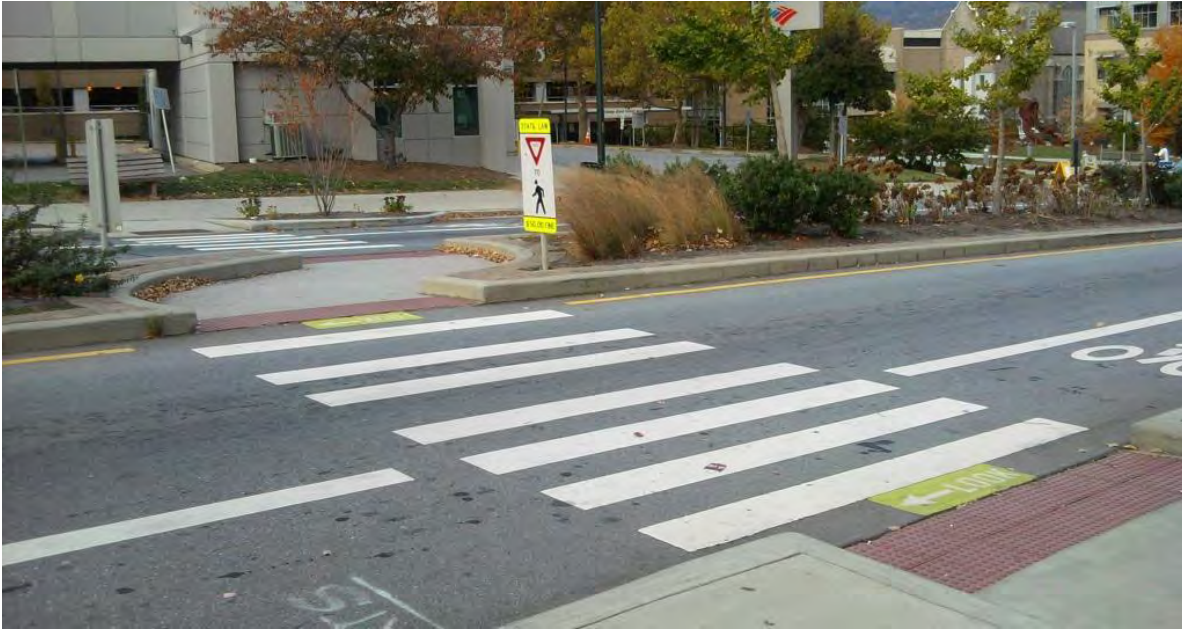
Figure 64: Pedestrian Refuge Island Example (Source: PEDSAFE)
