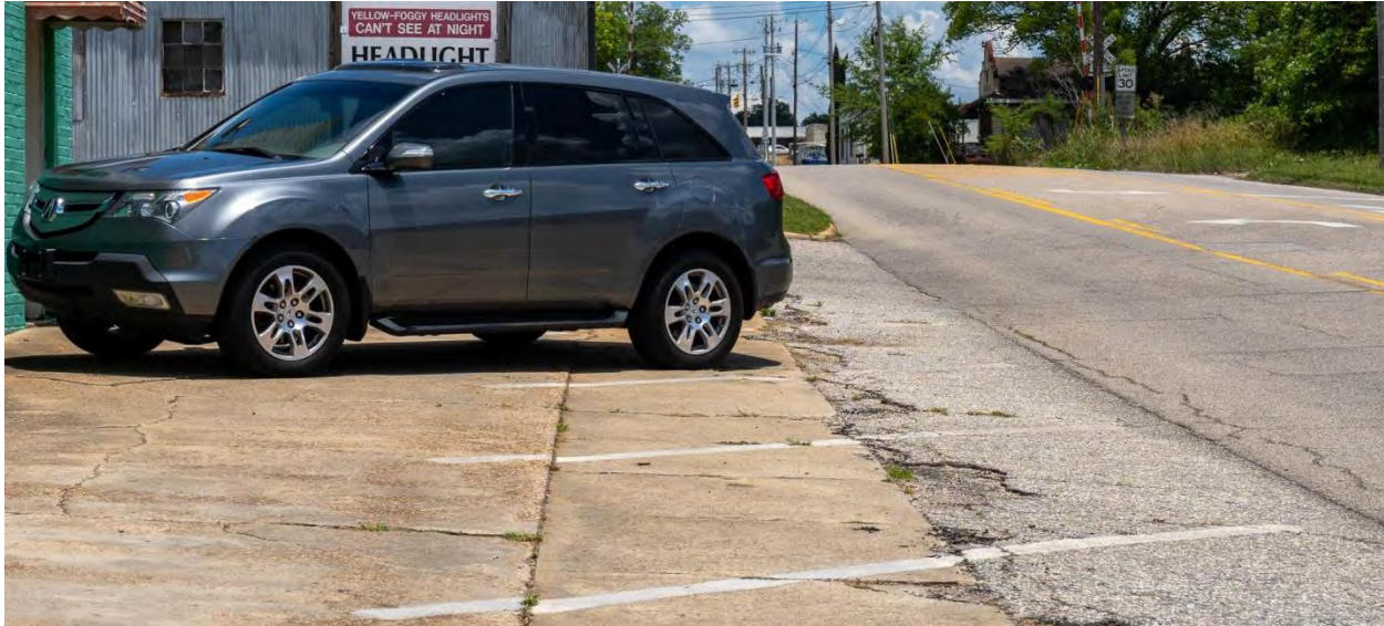
Photo 2: 1st Avenue sidewalk used as vehicle parking
