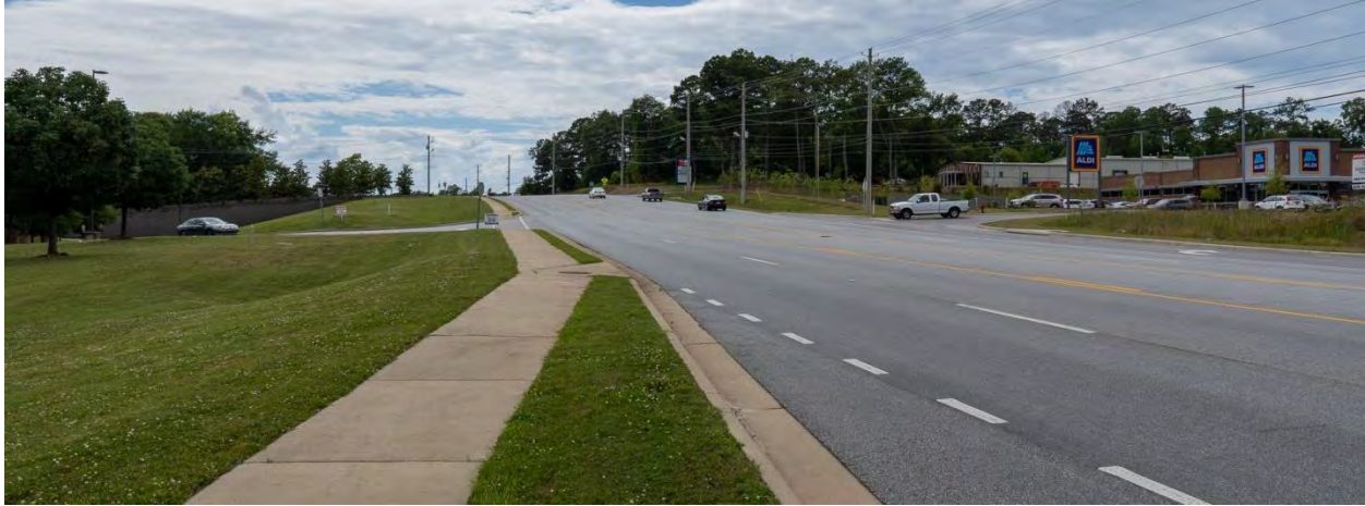
Photo 4: Sidewalk on the south side of Frederick Road near Tiger Town Shopping Center
