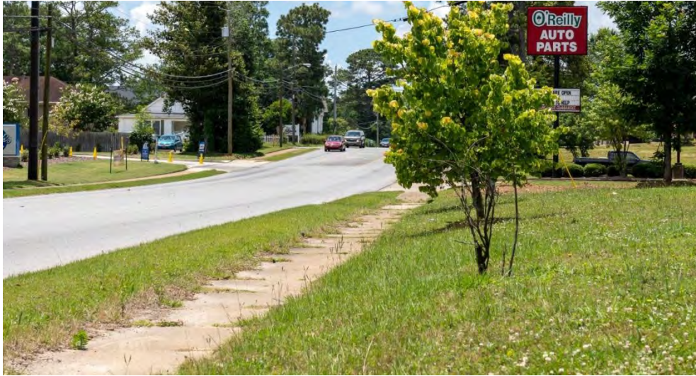
Photo 3: Existing Sidewalk along 2nd Avenue
