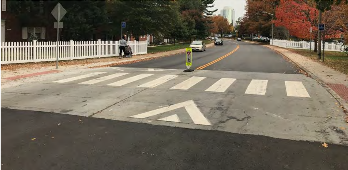
Figure 63: Example of Raised Crosswalk in Alexandria, VA (Source: PEDSAFE)
