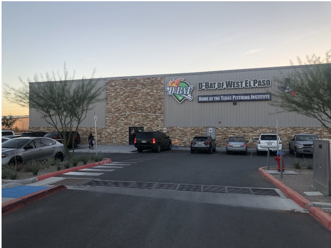
Photo of similar facility provided by the applicant.
