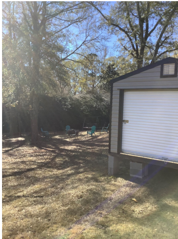
Photo taken near driveway & structure; concrete blocks leveling, 2 feet 4 inches high; Slope of Rear yard
