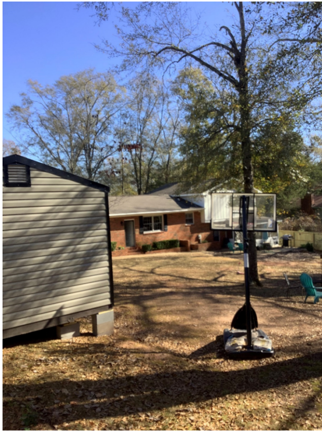
Rear wall of structure; leveling at structure corner; slope of rear yard area
