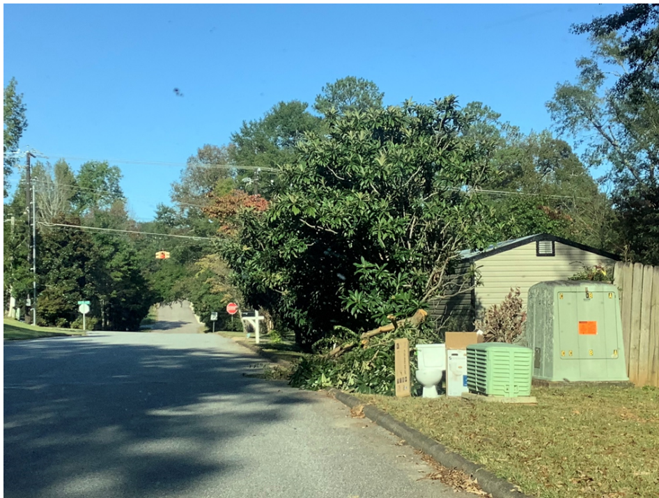
Photo from Northgate Drive toward Oak Bowery Road – Rear of Structure
