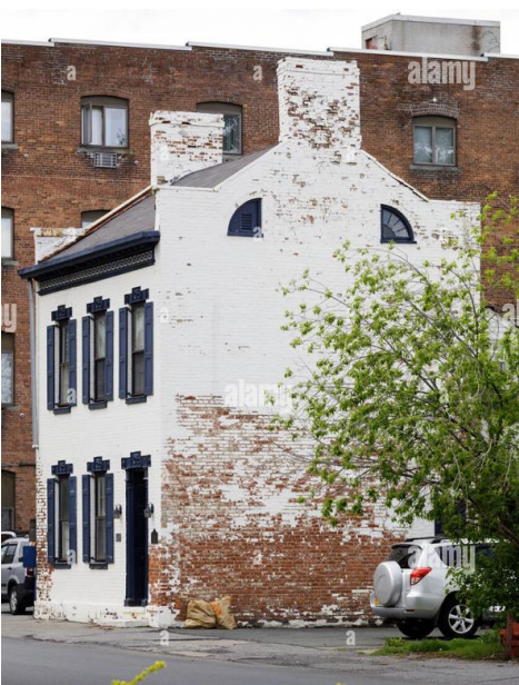
Federal bldg w/gabled parapet walls
