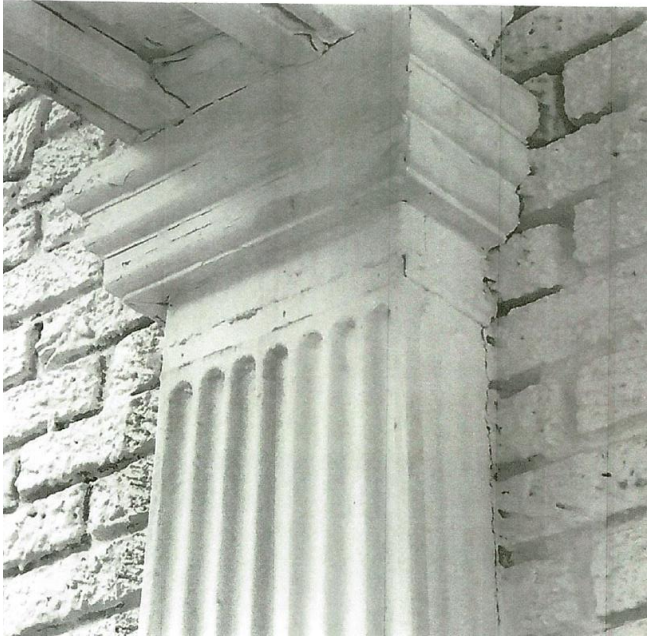
Details of pilaster on left elevation
