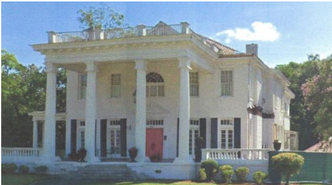
Right side porch removed
