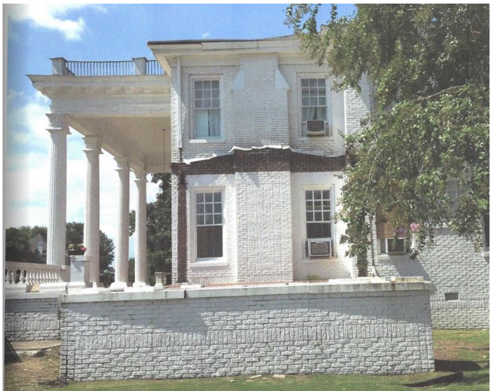
Right elevation to be repaired
